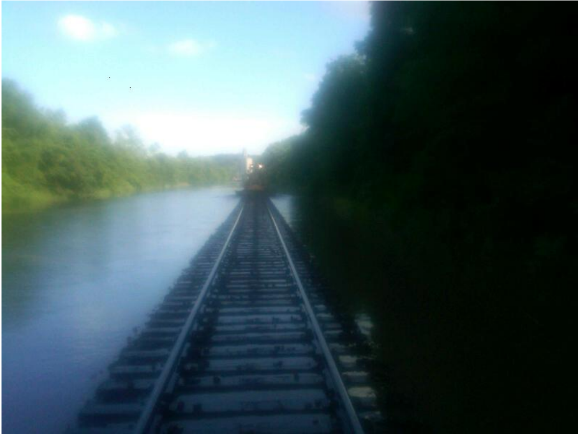
Falls City Sub
